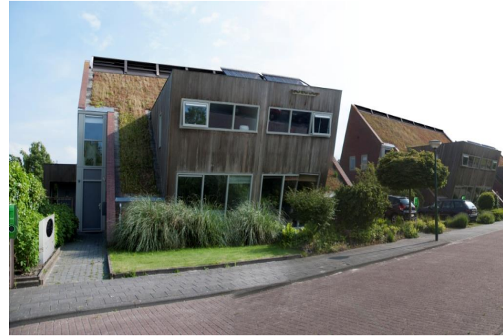
New housing Heeg with heatpipes, air water heat pump and roof ridge turbine
