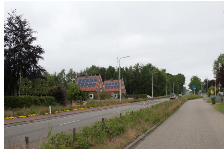
Huuskes with solar PV panels, roof ridge turbine and air water heat pump
