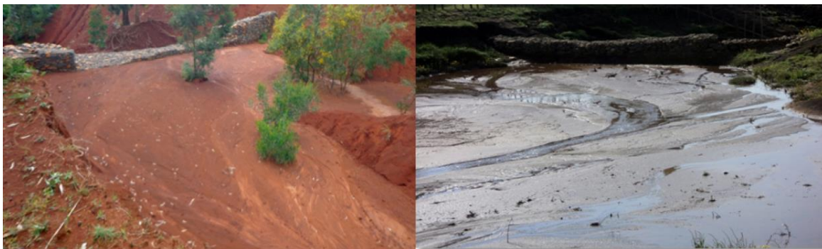
Figure 5.3 Example SSDs and trapped sediment at Segno Gebeya (left) and Enchet Kab (right) (Photo by Mulatie Mekonnen)
