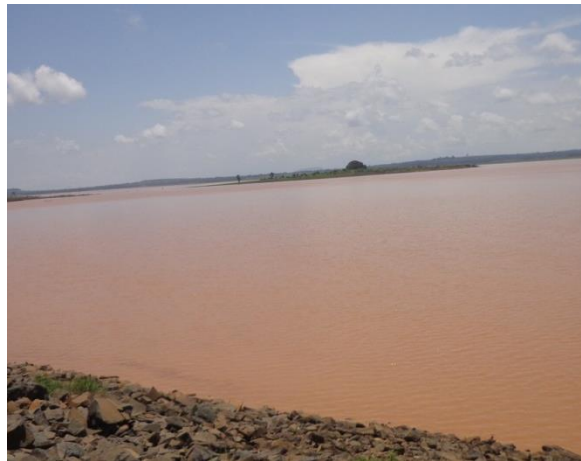
Figure 1.2 Koga reservoir with dark brown coloured water due to high suspended sediment concentration
