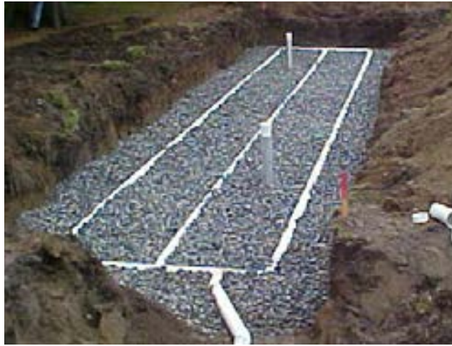
Figure 6.18 One example of the underdrained system consists of perforated pipes and gravel beds. Source: http://www.septicplus.com .
