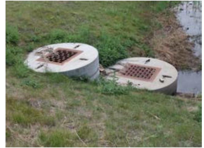
Figure 6.19 One example of the raised water outlet. Source: http://webpages.uidaho.edu .
