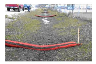
Figure 4 Installation of filter socks in a road ditch, Indiana, US. Source: Filtrexx International, LLC.
