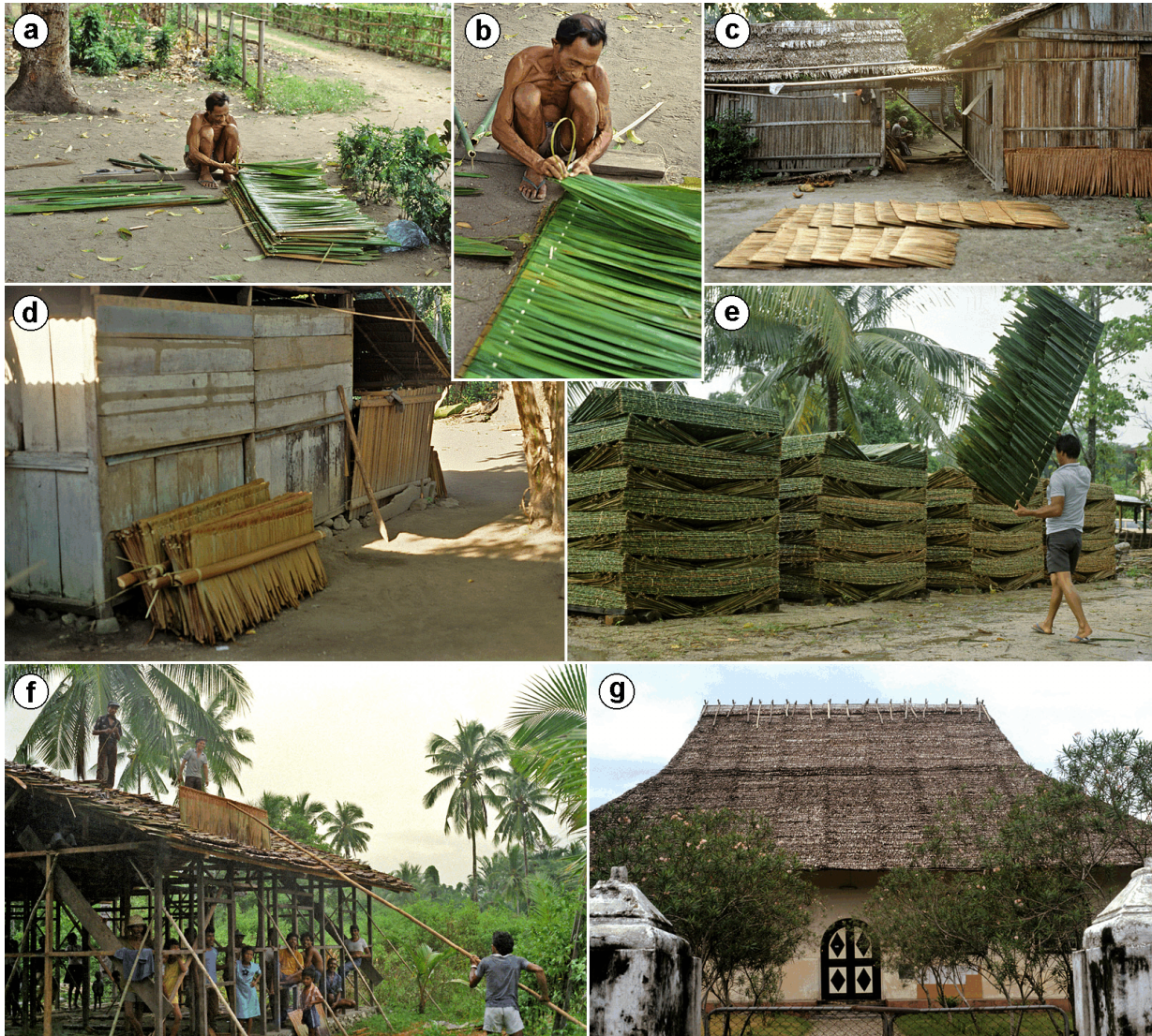
Figure 2.2 The main secondary use of the sago palm: the use of its leaflets for roof thatch ('atap'). a,b: Making 'atap sagu' shingles by folding leaflets over a lath of split bamboo culm and fastening them by sowing with a thin strip of split bamboo culm. [photo nrs 90.07-123-10 and -11, Hatusua, West Seram, Indonesia sun24jun1990] c: Drying sago leaflet shingles. In the background are houses with gaba-gaba walls and with roofs thatched with sago leaflet shingles. [photo nr. 88.12-074-05, Hatusua tue13dec1988] d: Home industry: two packs of sago leaflet shingles held together by lengths of gaba-gaba, ready to be sold. [photo nr. 90.06-122-13, Hatusua sun24jun1990] e: Small-scale industry: stacks of still green sago leaflet shingles. [photo nr. 86.03-II-31, N. of Batu Pahat, Johor State, Malaysia fri07mar1986] f: Putting up a sago leaflet shingle on a house under construction. [photo nr. 89.05-085-28, Hatusua sun14-mon15may1989] g: Church with roof cover of sago leaflet shingles. [photo nr. 89.08-093-26, Nolloth village, Saparua Island, Central Moluccas, Indonesia thu17aug1989]
