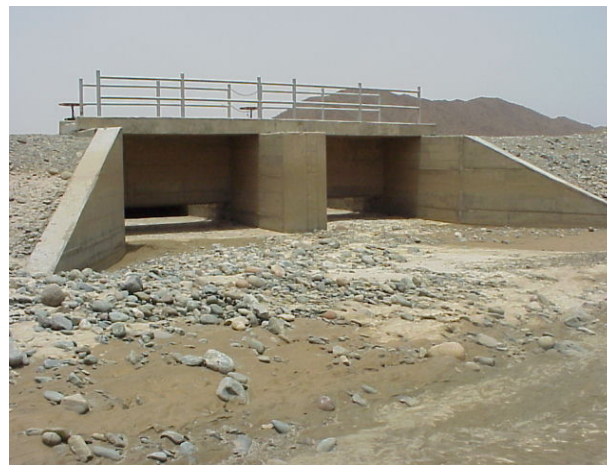
Figure 4.12 The Sheeb-Kethin culvert
