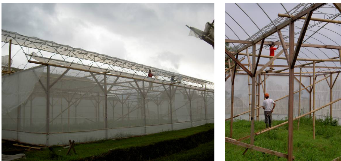
Figure 25. Construction of a modified Malaysian type plastic house.
