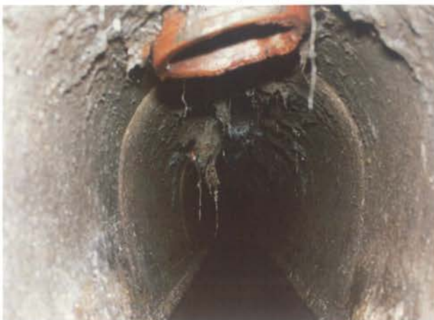
Domestic sewer connection with elliptical profile
