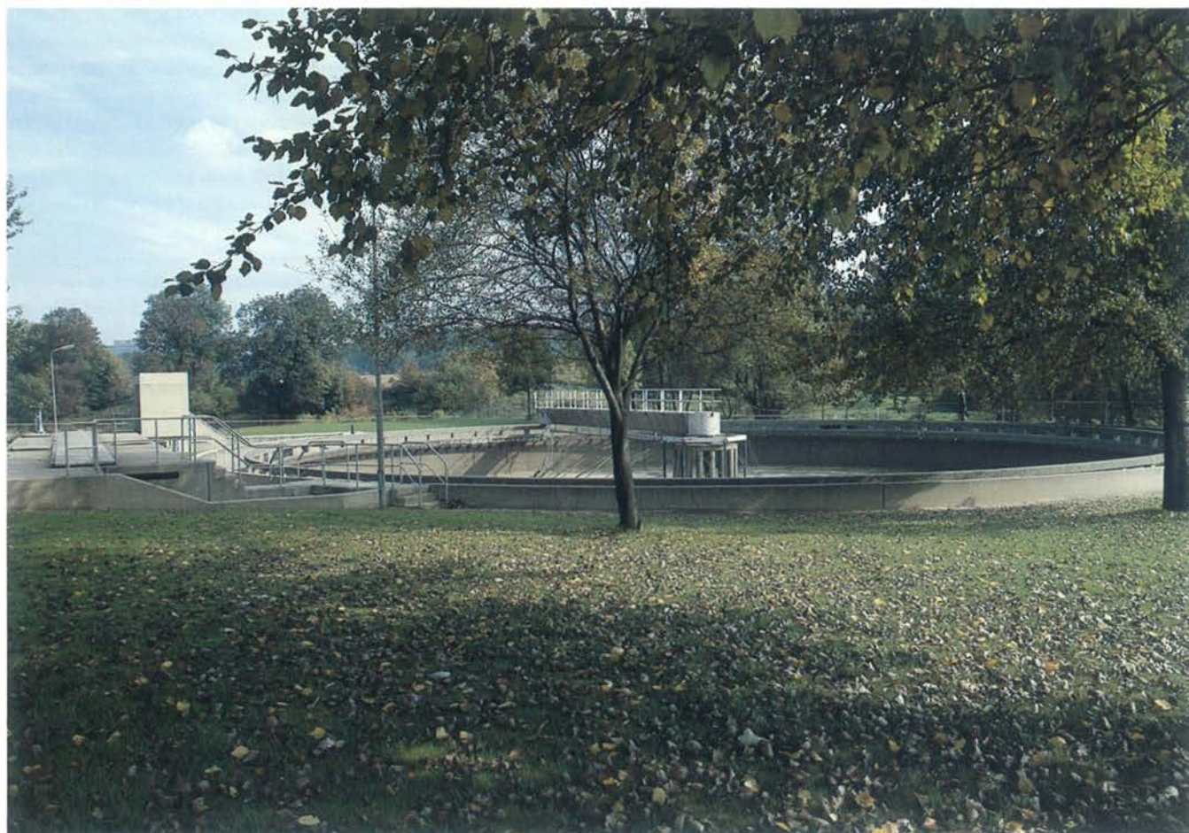
Stormwater sedimentation tank at Kerkrade
