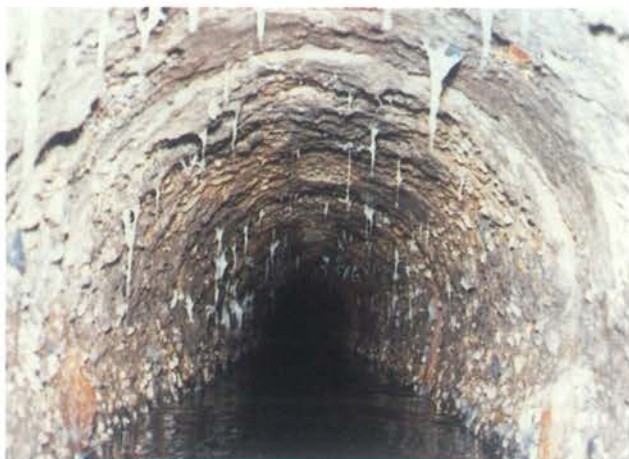
Deposits on the inside of a sewer
