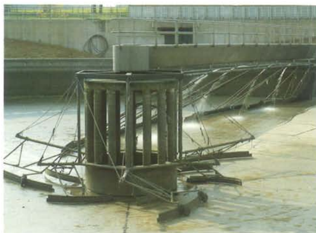
Stormwater sedimentation tank
