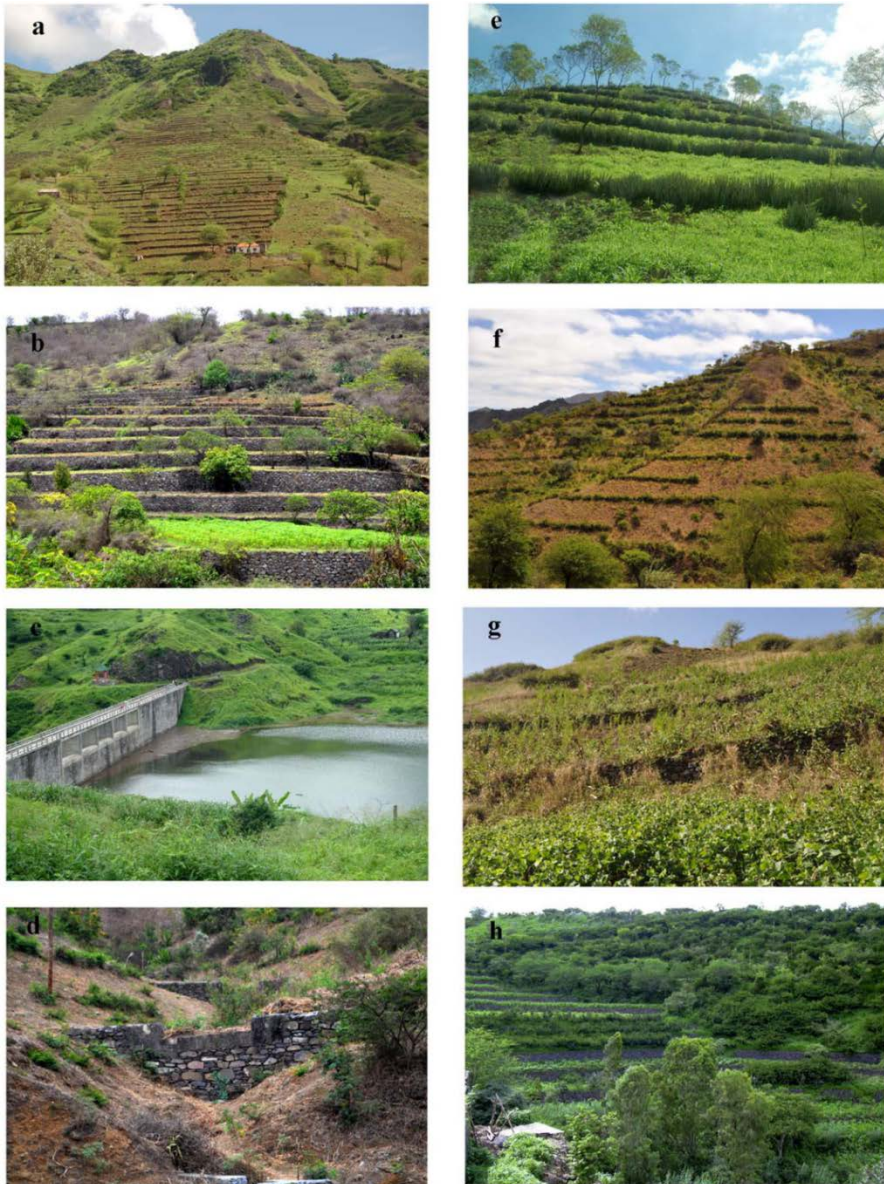
Figure 2.6 Vegetation and structural soil and water conservation measures in the Ribeira Seca Watershed: contour rock walls (a); terraces in São Jorge (b); Water collecting dam (Poilão) during rainy season (c), check dams on water ways in Godim (d); Aloe Vera barriers in São Jorge (e); L. Leucocephala hedges (f); Pigeon-pea on terraced fields (g); and Afforestation with different species in Longueira Baixo (h).
