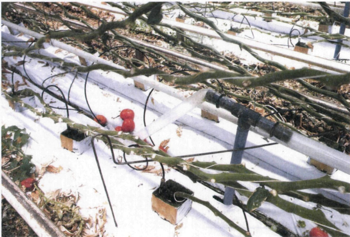
Distribution system for CO 2 with hoses pinched by stems or fruits because the pressure in the hoses is too low
