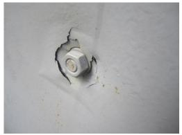
Picture 37. Broken epoxy paint by bending
