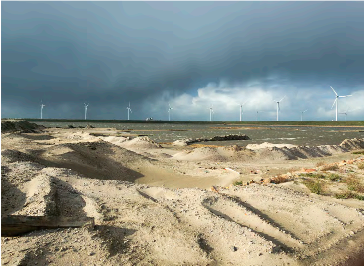
Second Maasvlakte under construction
