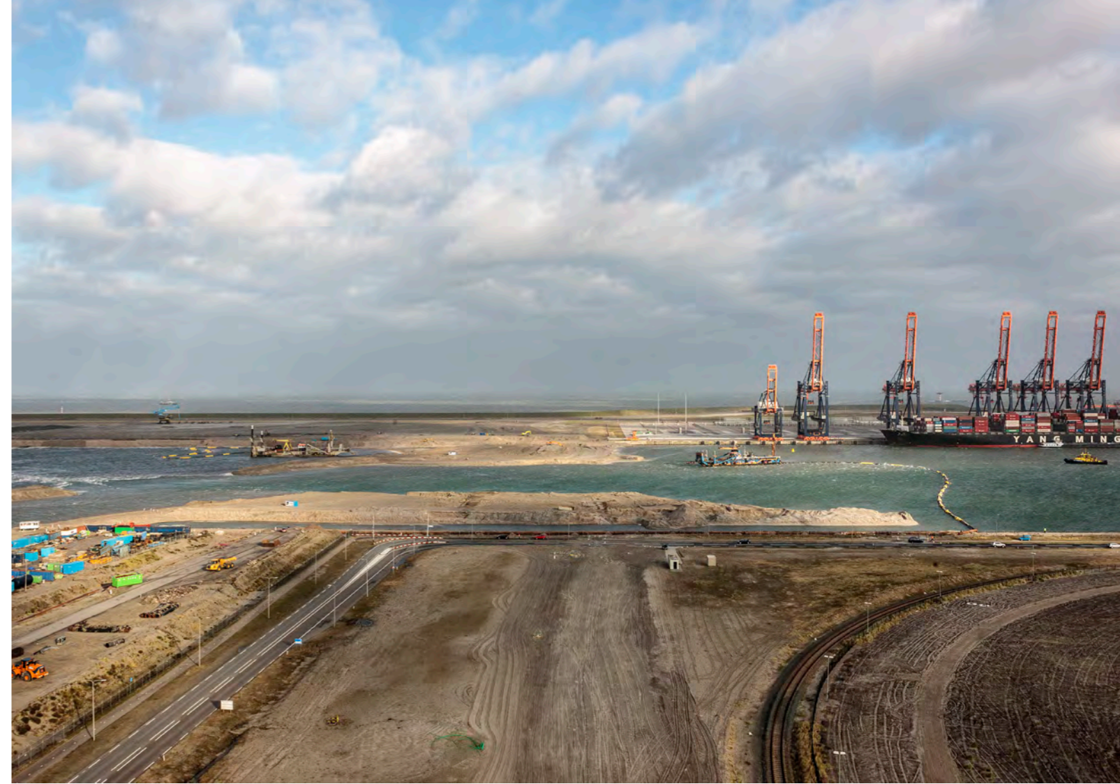
Second Maasvlakte under construction
