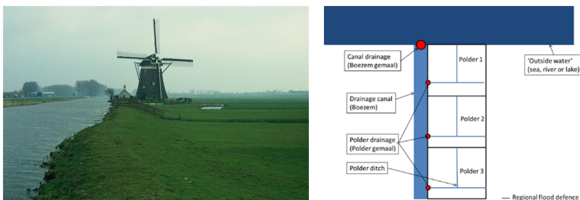
FIGURE 8 LEFT: TYPICAL STORAGE CANAL (RIJKSWATERSTAAT), RIGHT: SCHEMATIC VIEW OF POLDER, CANAL AND OUTSIDE BODY OF WATER
