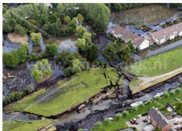
FIGURE 18: REGIONAL FLOOD DEFENCE BREACH AT WILNIS, 2003 (SOURCE: KOENSUYK PHOTOGRAPHY)
