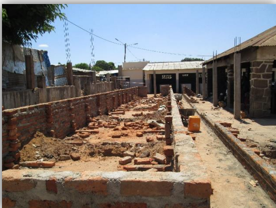
Picture: Construction of new shops on the Manica market.
