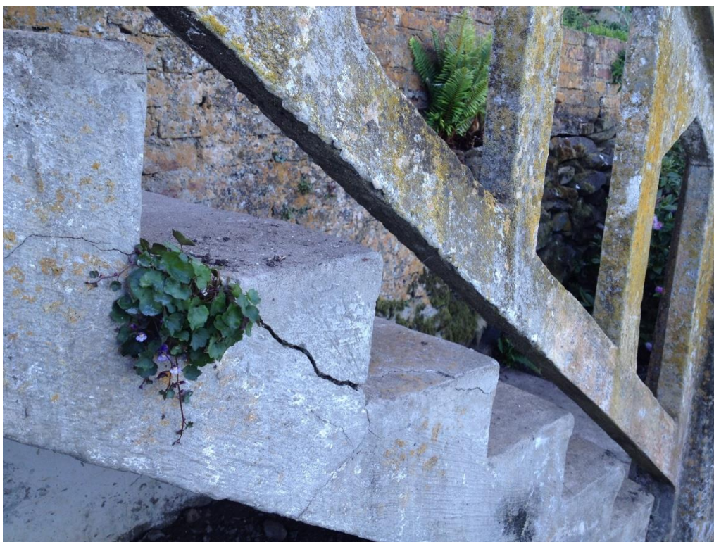
Figure 9. Stairs built during the rehabilitation project. Kenilworth ivy, which grows out of hard surfaces all over the island, can be seen growing from a crack. Whether the ivy is causing the crack, or taking advantage of it, is hard to tell (Photo by author).
