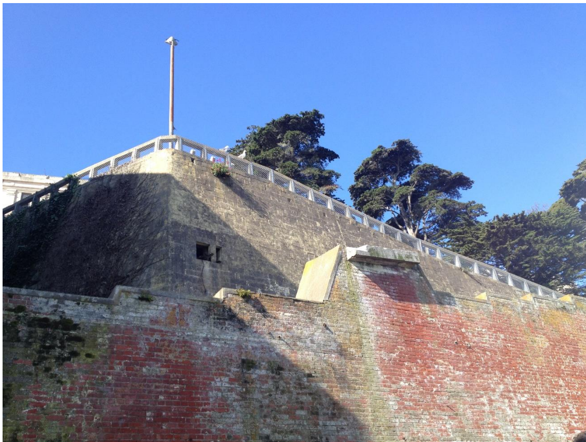
Figure 5. Perspective on Alcatraz's layered history. The bottom layer shows brick that was the main material of the military era. Above this are concrete blocks from the penitentiary era, both topped off by a canopy of Monterey cypress (Photo by author).
