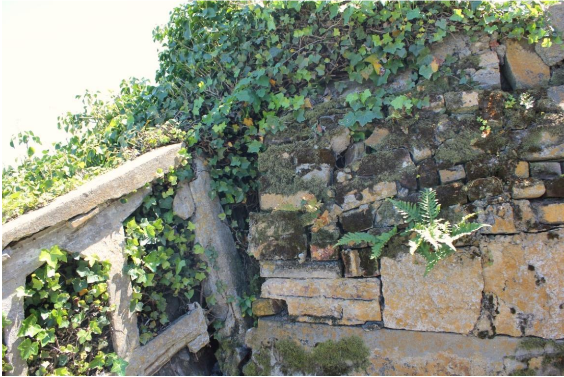
Figure 19. This ivy has been growing here for so long that some of the interior crevices of this concrete railing have become filled with thick, woody stems (Photo by Llessica Chan).
