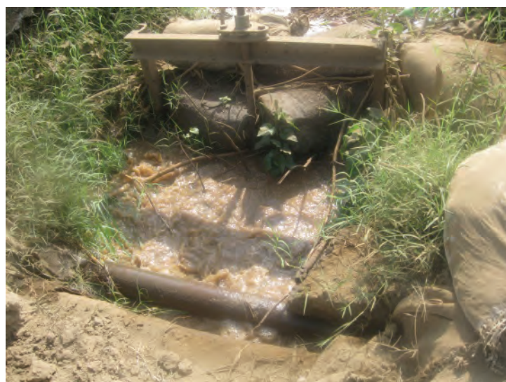
Figure 5.41. Sacks and grass used by farmers to control the water delivered to Gemoia Minor Canal
