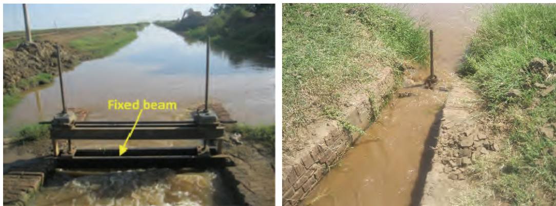
(a) Fixed beam at the movable weir
