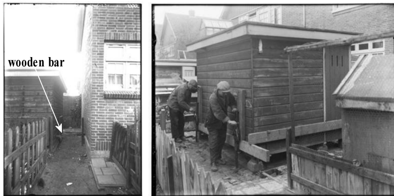
Figure 4.8: Left: difference in ground settlement between a structure with (brick house) and without (wooden shed) a piled foundation. The wooden bar indicates the level of the base of the shed after construction. Right: people jacking up a shed. Photographs taken in 1935.
