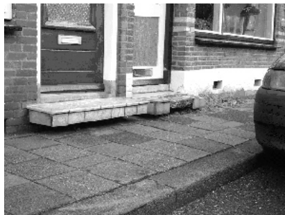
Figure 4.2: Creative solution to allow for entrance after ground settlement.
