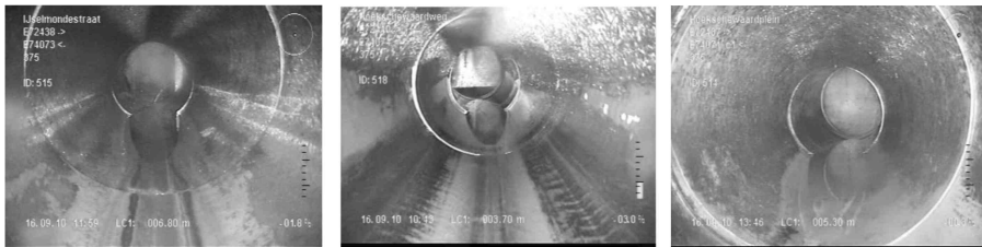
Figure 5.11: Photographs of hinge sewers made of PVC and constructed in 1997 showing small sags just in front of the manhole with a deep foundation.
