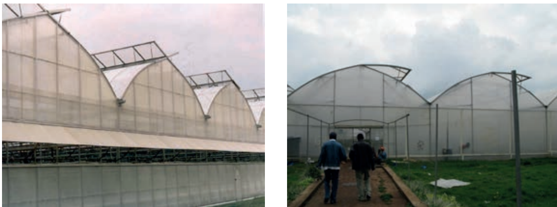
Figure 3.4 Natural ventilation (two-side, one-sided).
