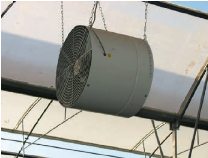
Figure 3.6 An air circulation fan can stimulate air movement in a greenhouse.
