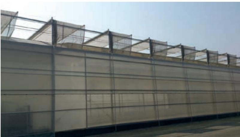
Figure 3.9 External shading screens (mid-tech greenhouse in Taiwan).
