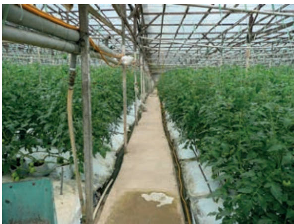
Figure 3.1 A greenhouse construction of local wood may be cheap, but is less durable and has lower light transmissivity than a aluminium greenhouse construction.
