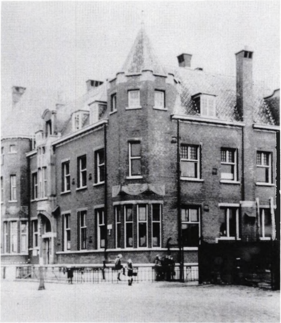
Fig. 9. The building at Eemskanaal ZZ 1 in Groningen, where the 4th and 5th departments of the experimental station were housed.
