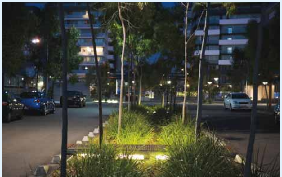
Bioretentie van regenwater in Victoria Park in Sydney (foto: Tony Wong).
