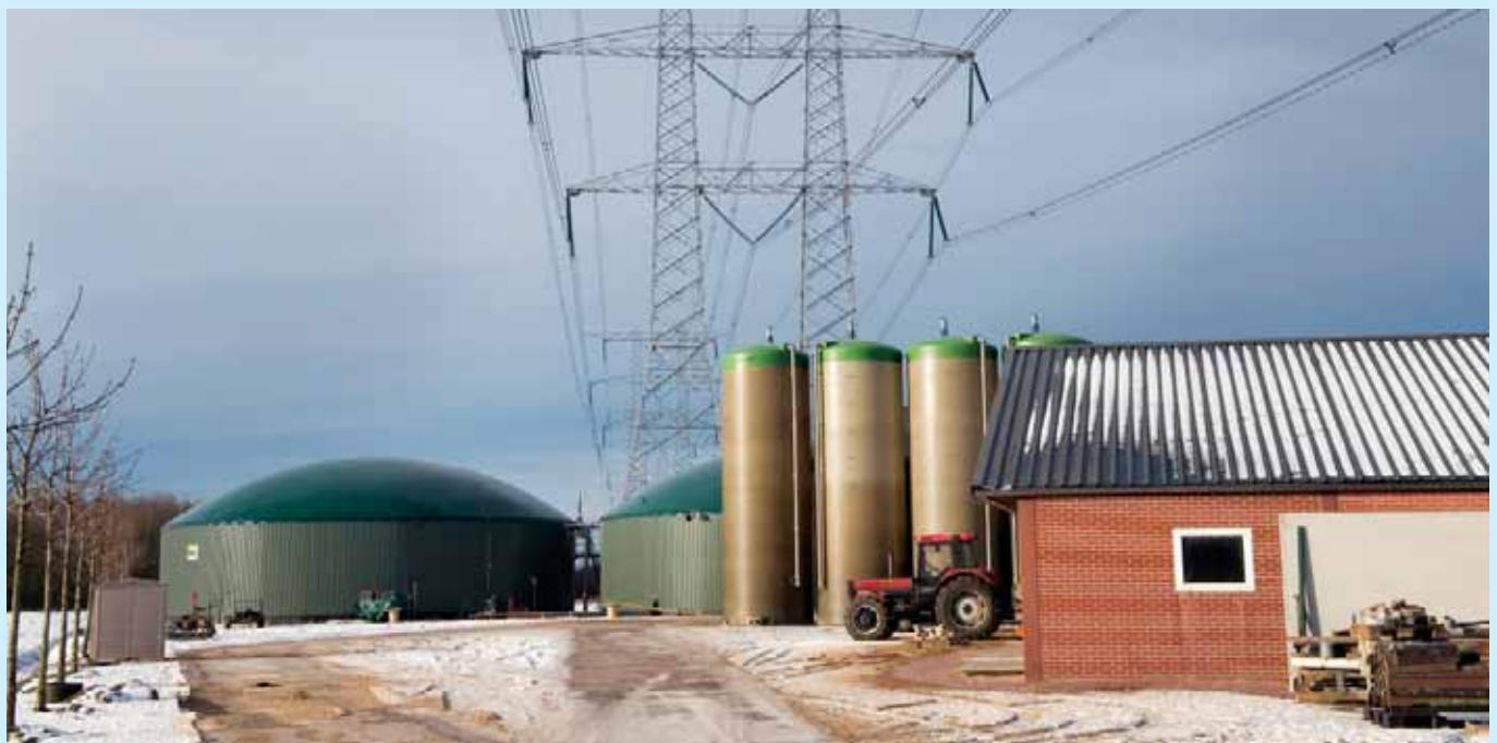
Biovergistingsinstallatie in Bakel.
