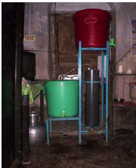
Figure 6.3 A third generation UNESCO-IHE Family Filter installed in a village in Bangladesh.
