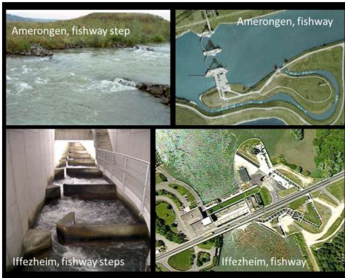
Figure 3.3. Photographic impression of the fishway steps at Amerongen (top left) and Iffezeheim (bottom left), and top views on the fishways at Amerongen (top right) and Iffezeheim (bottom right). The fishways at Hagestein and Driel are very similar to Amerongen. The fishway at Gambsheim is very similar to Iffezeheim.
