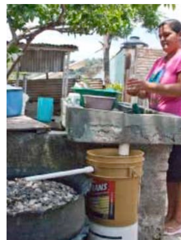
Image 5. Greywater filter adaptation. Source: (FAO, 2012a)
