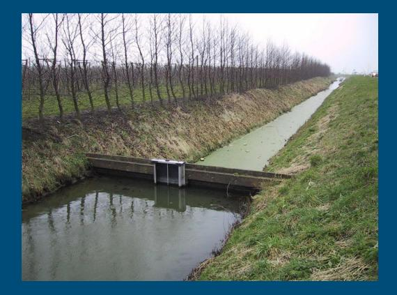
a water conveyance system that receives water from the field drainage systems, surface runoff, and groundwater flow, and transports it to the outlet point
