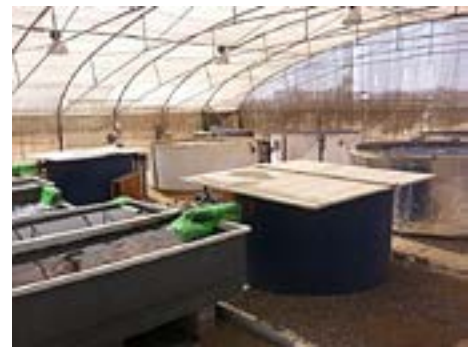
Overview of the fish unit with round fish tanks at the back and clarifiers at the front (Photo: Ziad Abu El Nasr)
