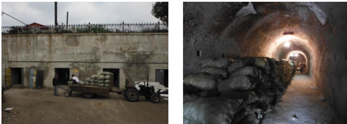
Figure 5.1. Front view of tunnel stores (left), tunnel store (right).
