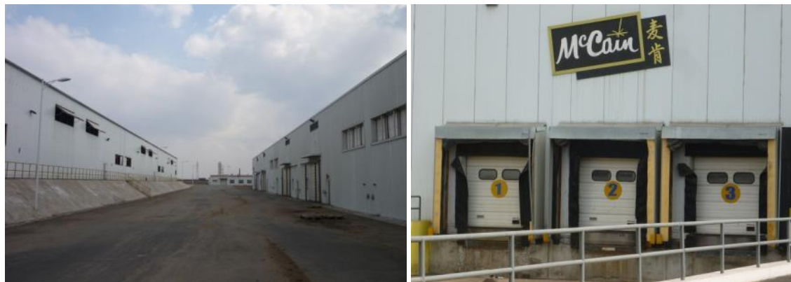
Figure 5.4. Pictures of McCain storage facility in Harbin (April 2014).
