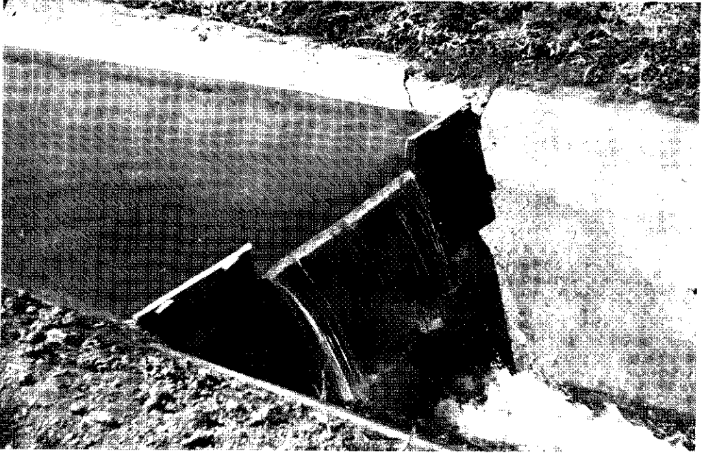
Photo 1. Rectangular sharp-crested weir.
