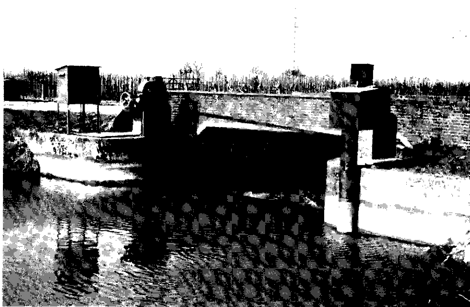
Figure 1.9 A broad-crested weir with movable crest can be used to regulate and measure the flow into a canal. This combination of functions facilitates the control of irrigation water.
