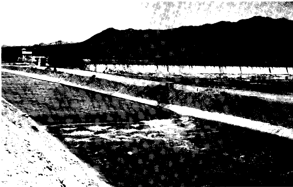
Figure 1.6 This 15.45 m wide flume has a throat length of 3.05 m. At its design capacity of 56.6 \text{ m}^3/\text{s} , a head loss of only 0.12 m is required for flow to be modular. On large structures, a 1-to-6 downstream ramp reduces construction cost. Low crests ( < 0.5 \text{ m} ) often have a vertical downstream face.
