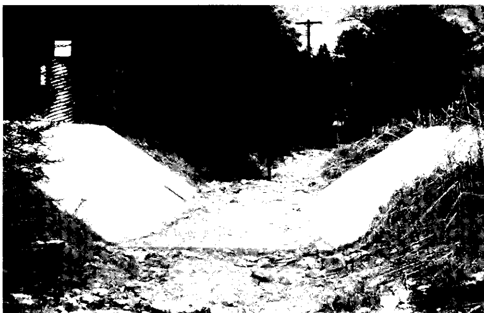
Figure 4.7 Flat-bottomed long-throated flume in sediment-transporting stream. Has been operating since 1970
