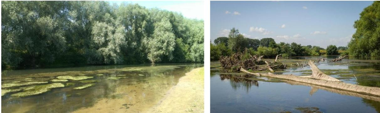
**Figure 12-15 Large restoration project DL\_R1. Upstream view of the widened and shallow cross-section (left) and large wood placement (right) (UDE)**
