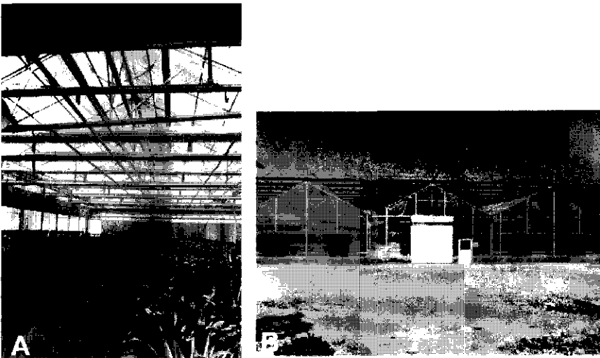
Fig. 6.5: (A) Outside and (B) inside view of a modern Chinese-made polycarbonate greenhouse near Jinan equipped with a pad-and-fan cooling system and an external screen.
