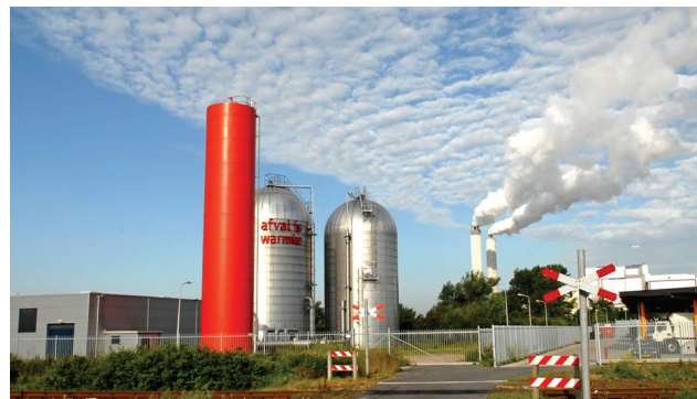
Figure 5.5 Heat storage tanks of AEB. Text on the tanks says: "waste is warmth". Source: www.noord.amsterdam.nl
