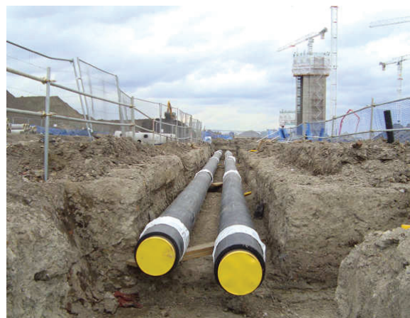
Figure 5.21 A district heating- and cooling network in construction. It exists if insulated tubes filled with a liquid as thermal energy carrier. Source: www.ceequal.com .
