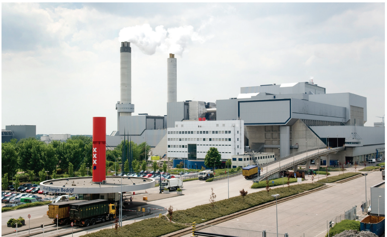
Figure 5.7 AEB located in the port of Amsterdam processes waste into electricity and district heating. Source: www.nieuwsbrief.amsterdam.nl
