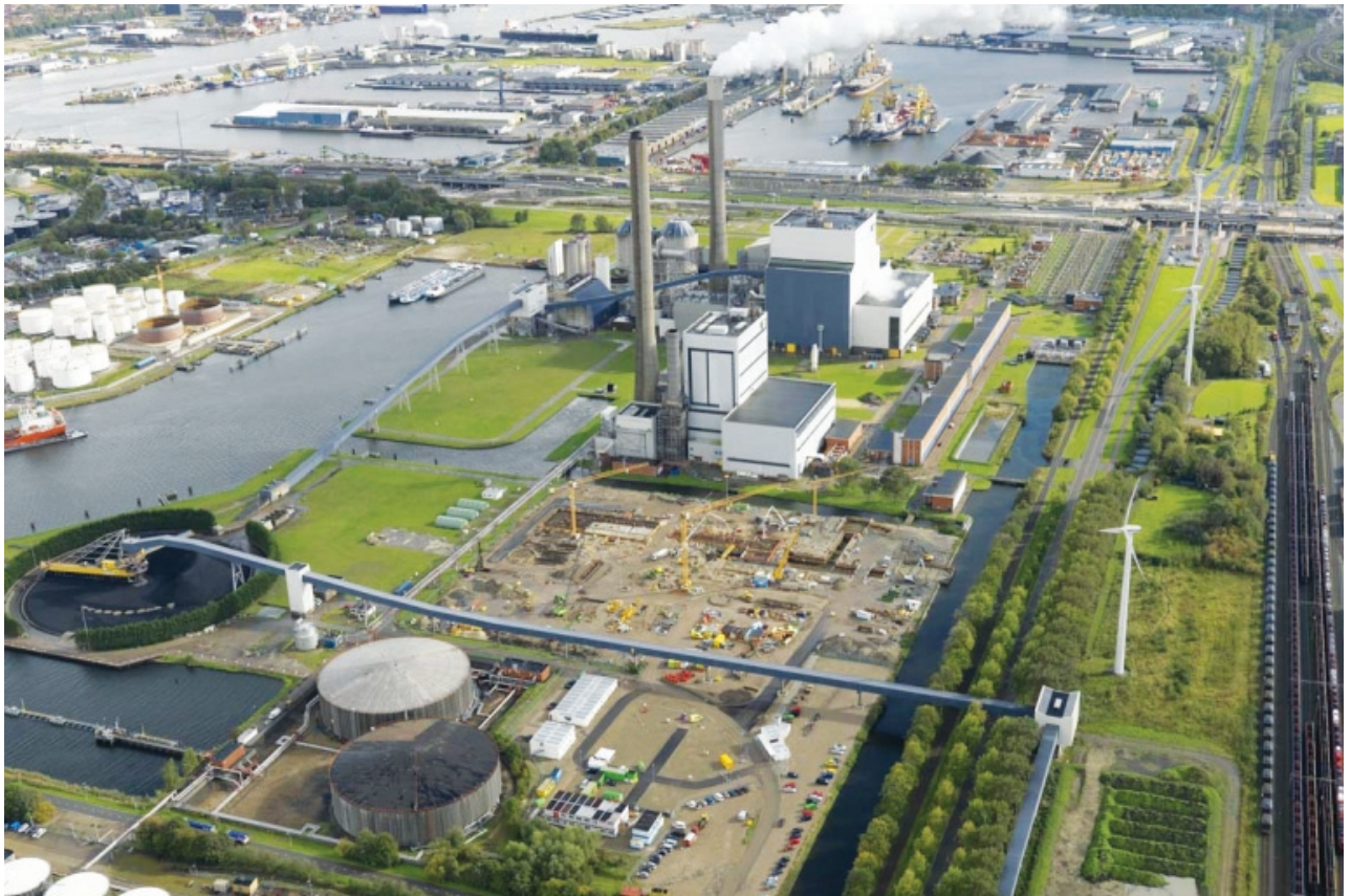
Figure 5.6 The power plants Hemweg supplies electricity by means of coals and natural gas. It's residual heat however is disposed into the air, while it has potential for district heating. Source: www.kecpro.com .
