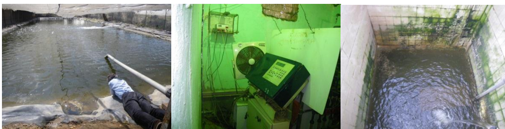
Figure 17-19: The water basin, HortiMaX fertigation control and drain water collection
