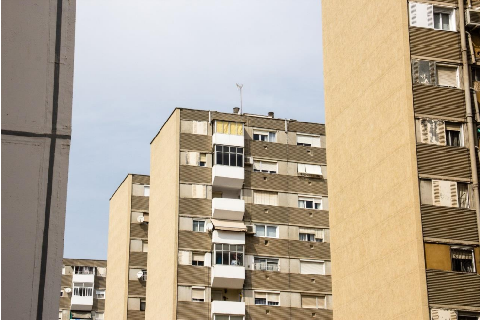
Image 20: Deterioration of buildings (1)
