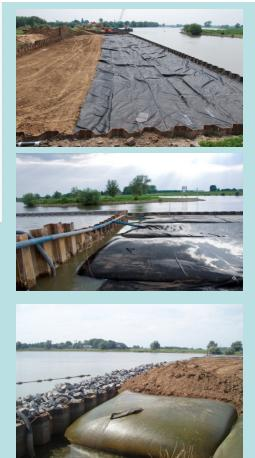
sustainable riverbank-recovery in Zutphen near river IJssel - 18.000 tons sediment, 450 meters
