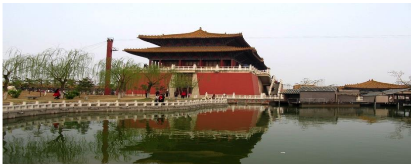
Figure 7. City Gate Wall in QRLG.
