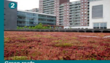
2 Green roofs Green roofs absorb rainwater, provide insulation and help to lower urban air temperatures. The Hague frantically promotes green roofs.
