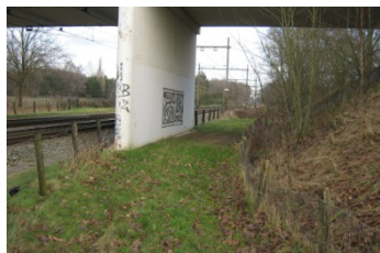
Foto 17 Viaduct over spoor (RL)
