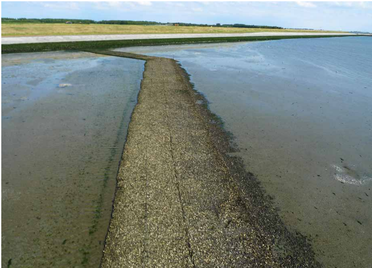
Figure 4 Oyster reef functioning as a breakwater and sediment stabilizer.
