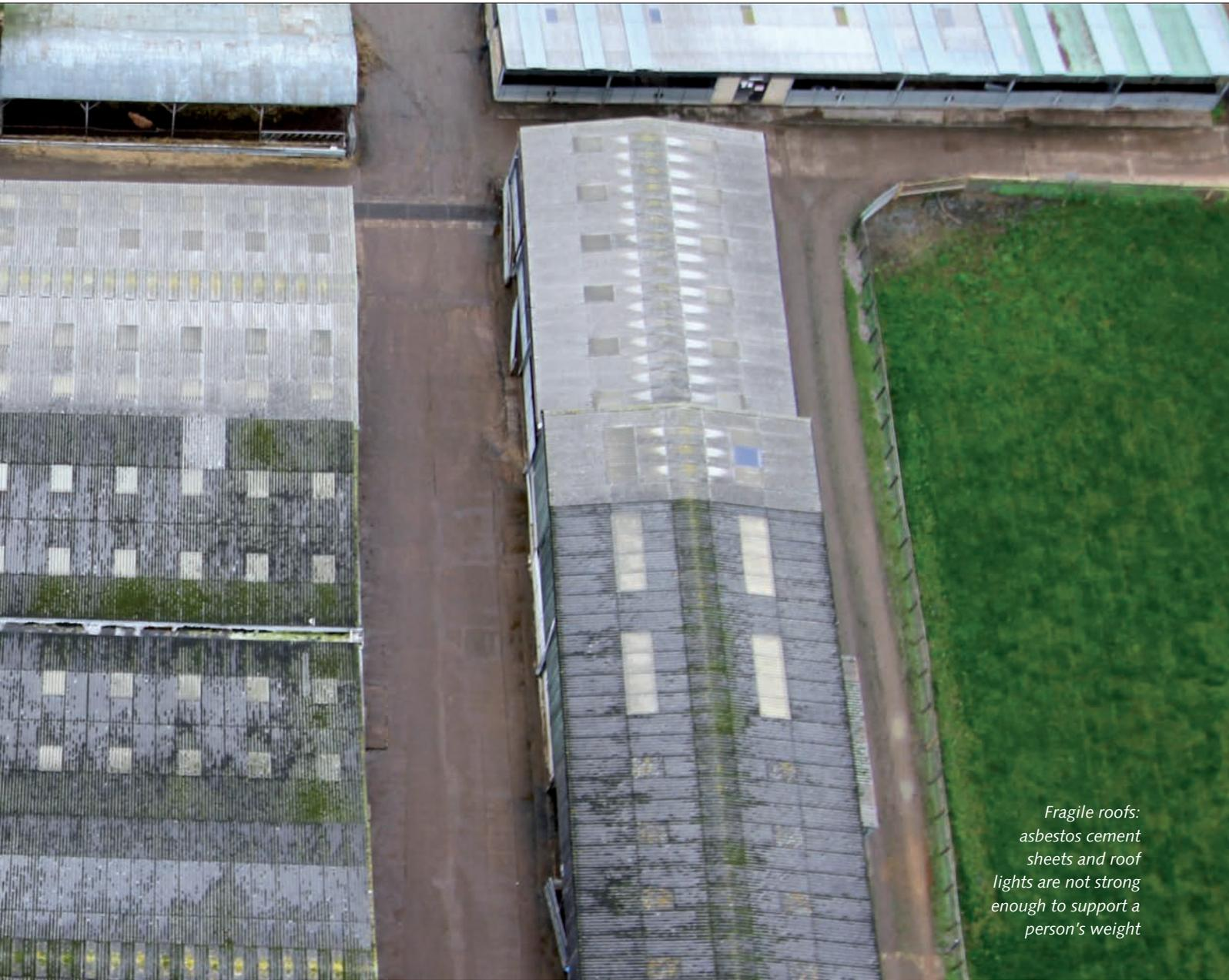
*Fragile roofs: asbestos cement sheets and roof lights are not strong enough to support a person's weight*
