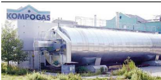
Horizontal plug-flow digester
