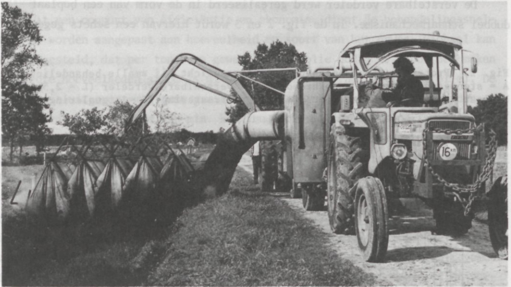
Fig. 4. The improvised steam treatment combination, arranged over a water course of average width.
