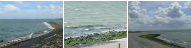
Picture 6.12. Dike failure, and the waves showing the relief and foams in old dike. Picture 6.13. and 6.14. show the relief of the renewed dike, with softer endings
