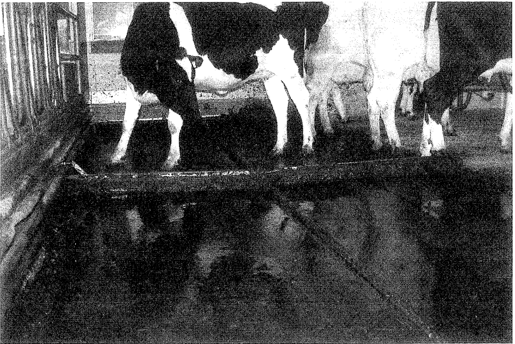
Solid concrete floor, sloped in a V design 3% to the centre, with a urine drain in the centre.
