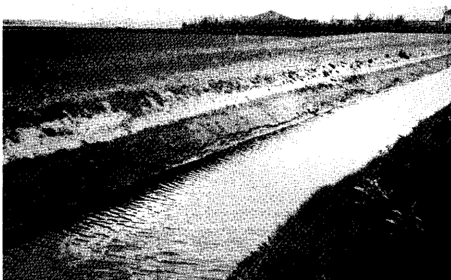
Fig. 25. Capillary moisture front on the freshly cleaned slope of a ditch (early summer 1976).
