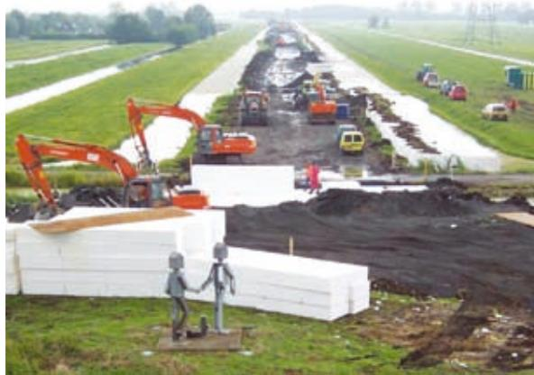
Figure 39: Building a road on EPS (polystyrene)
