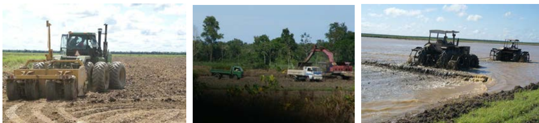
Figure 10 Levelling by scraper (left), hydraulic excavator (centre) both followed by puddling (right).
