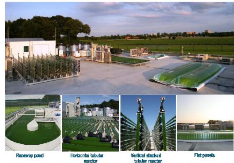
Figure 4 AlgaePARC. The opening of this facility took place in June 2011. There are 4 different production systems of 24 m 2 each and 3 of 2.5 m 2 each.
