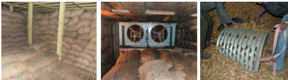
Figure 2. Some impressions of a traditional cold store with jute bags (left) and a cooling system at the top floor (centre) and an example of an upgraded cold store with bulk storage with forced ventilation (right).
