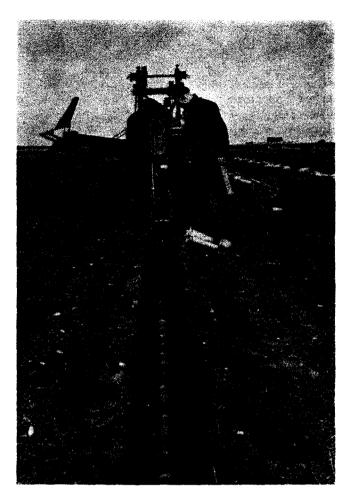
Fig. 13. A drainage machine replacing the provisional system of field ditches with tile drains.
